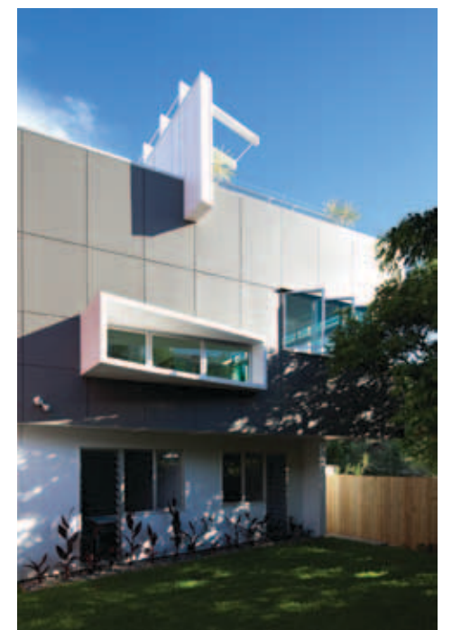
The entire north wall is angled to preserve the neighbours’ view, and also acts as an eave to protect the downstairs bedrooms from the summer sun. An angled surround gives privacy to the low living room window. The grey CSR Cemintel ExpressWall cladding is lightweight and quick to install.
