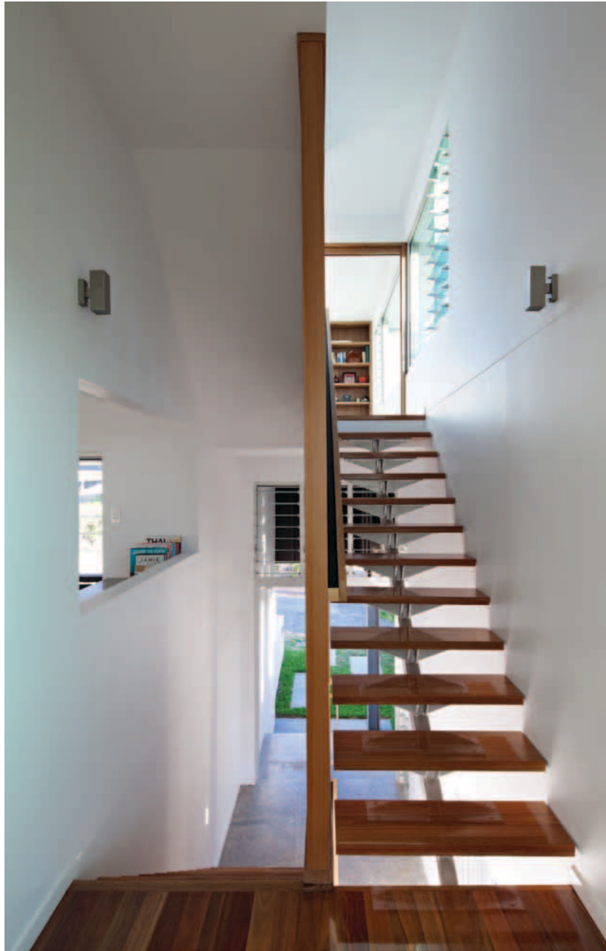
Open stairwells and an open layout without hallways allow maximum airflow through the house. The stair treads are supported by steel mono-stringers with steel brackets.
